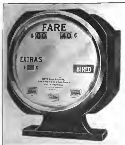
Fig. 4—Front view of Taxameter showing fare and extra register in service
